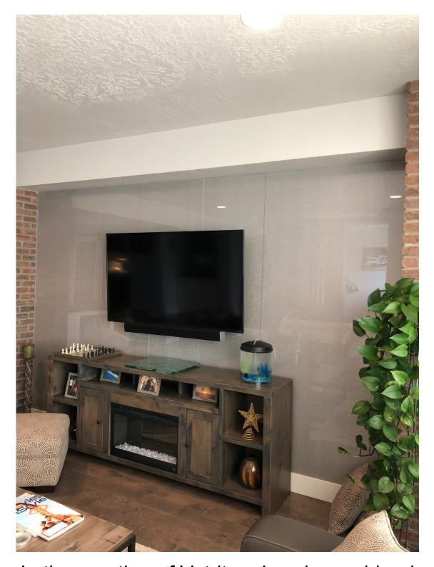
In the creation of Vetrite, glass is combined with fabric and polymeric film to create a profound material.
